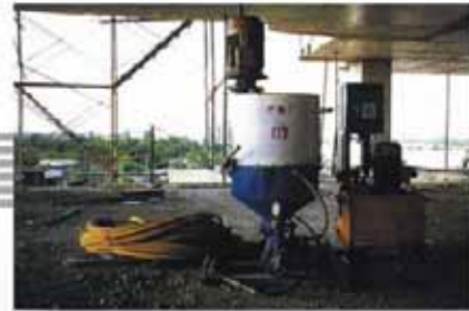
MODERN COLLOIDAL GROUTING MACHINE FOR EFFECTIVE GROUTING OF TENDONS TO ENSURE BOND AND CORROSION PROTECTION
