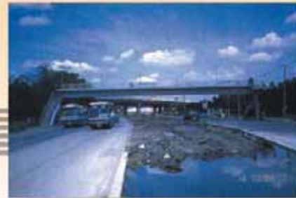
COMPLETED 36.00 M SPAN POST TENSION GIRDER FOR STANDARD PEDESTRIAN BRIDGE
