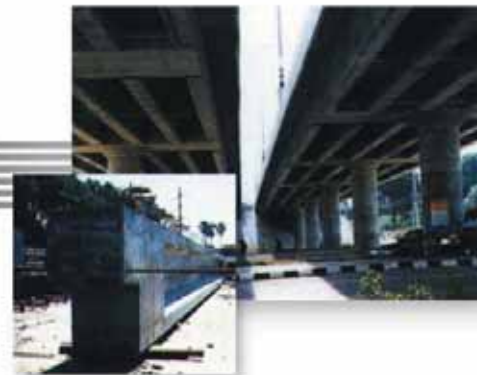
STANDARD HIGHWAY GIRDER 30.00 M. SPAN
