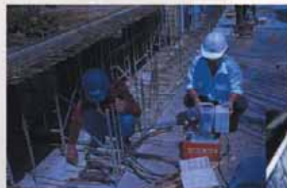
STRESSING OF PBL SUPER FORCES TYPE SF 405 BY MONO STRAND JACK V16
