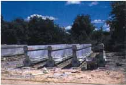
POST TENSION GIRDER PC 8801, 8802 FOR STANDARD HIGHWAY PEDESTRIAN BRIDGE
